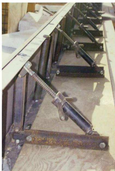
EDGE OF DECK FORMS
